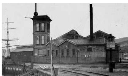
By the early 1880s, the city was beginning to grow to the extent that the background of houses behind the Customs House (STOP 1) reduced the visibility of the time ball. A new location for the time ball took some time to be agreed and finally in the late 1880s Shed J, a timber store, was built with a tower on which the time ball installed.
